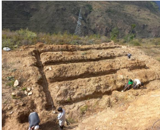
Figure 2. Foundation of smart greenhouse
