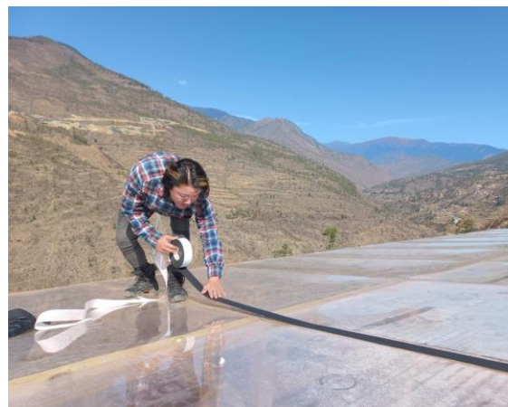
Figure 5. Sealing of leakages in smart greenhouse
