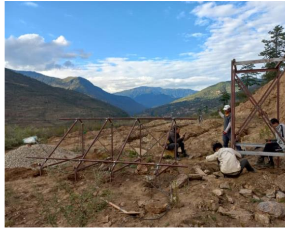
Figure 3. Structure component of Solar water heating system
