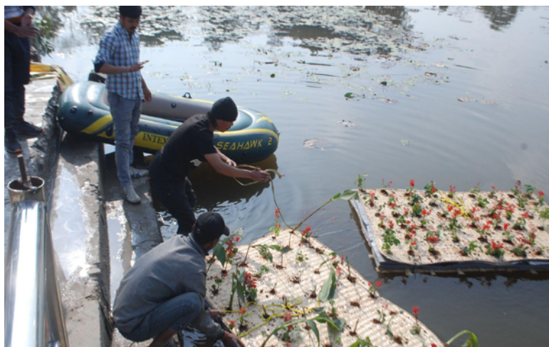
Figure 10: Raft installation (Picture credit: Samyak Prajapati, SEN)
