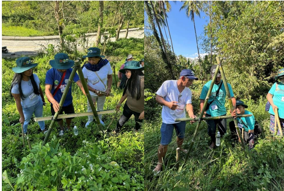
Figure 5-6. Participants from Barangay Tala ( left photo ) and Barangay San Cristobal ( right photo ) conducting contour line determination using A-frame.
