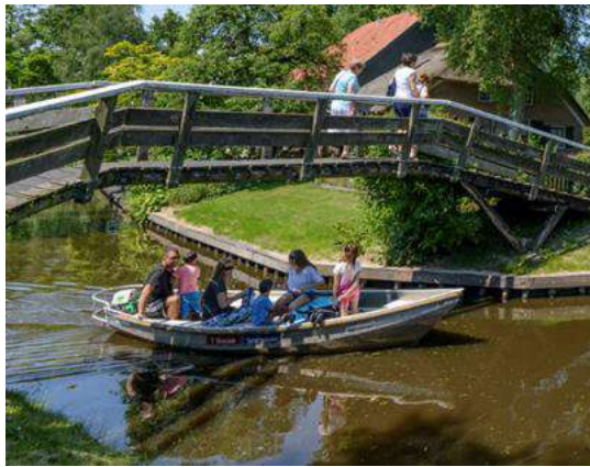
Figure 16: Water system in wetland park
