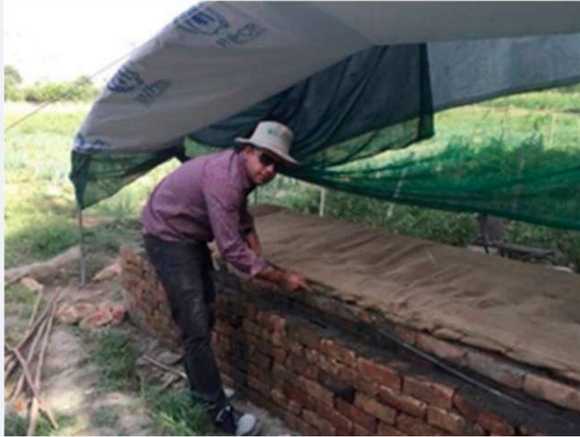
FIGURE 12. Zero energy cool chamber (ZECC), constructed by Amity University at Kabul University.
