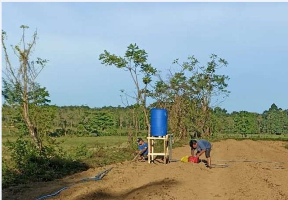
FIGURE 10. Connecting water source.
