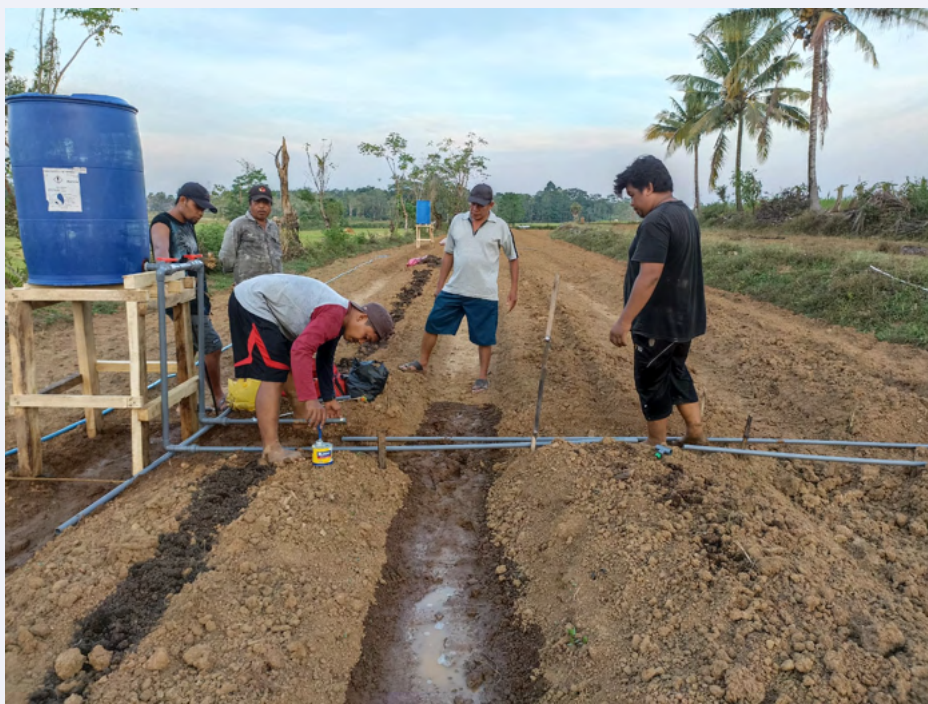
FIGURE 11. Connecting lateral pipes.
