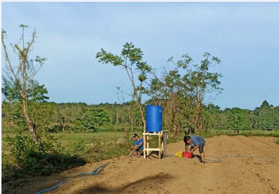
FIGURE 10. Connecting water source.
