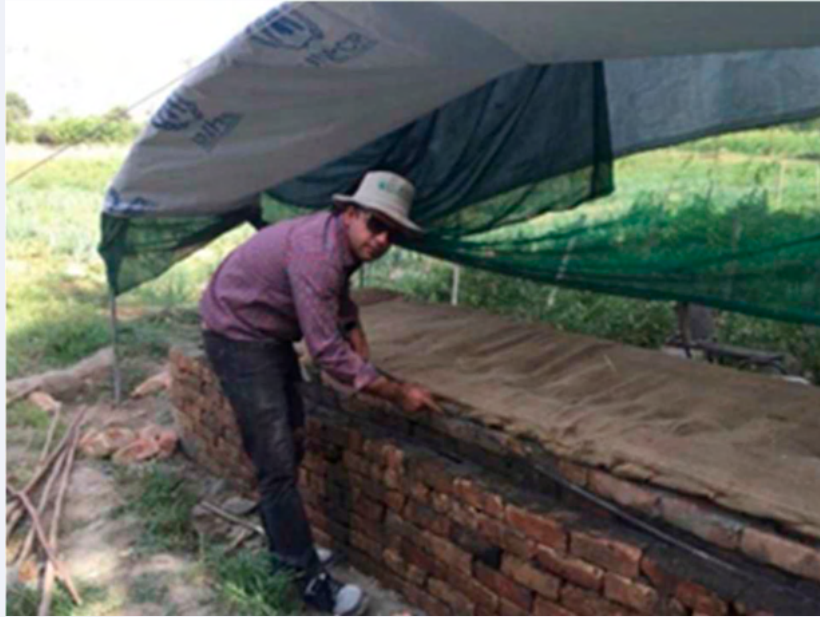
FIGURE 12. Zero energy cool chamber (ZECC), constructed by Amity University at Kabul University.
