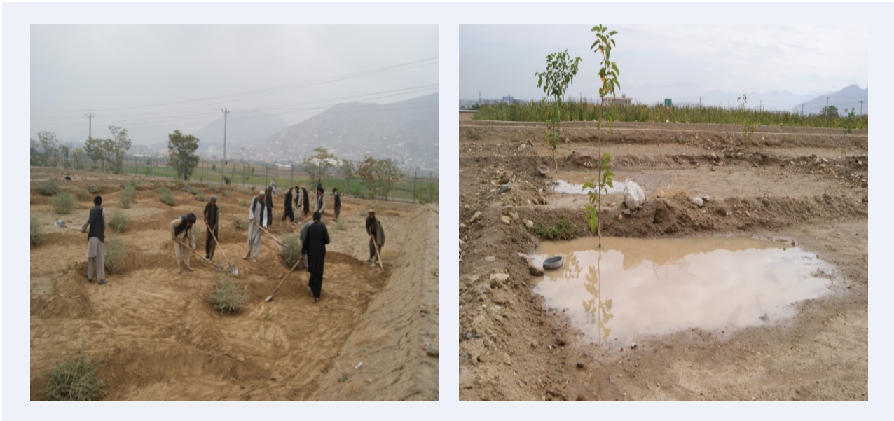
FIGURE 15. Rainwater harvesting using eyebrow pitting in Afghanistan.
